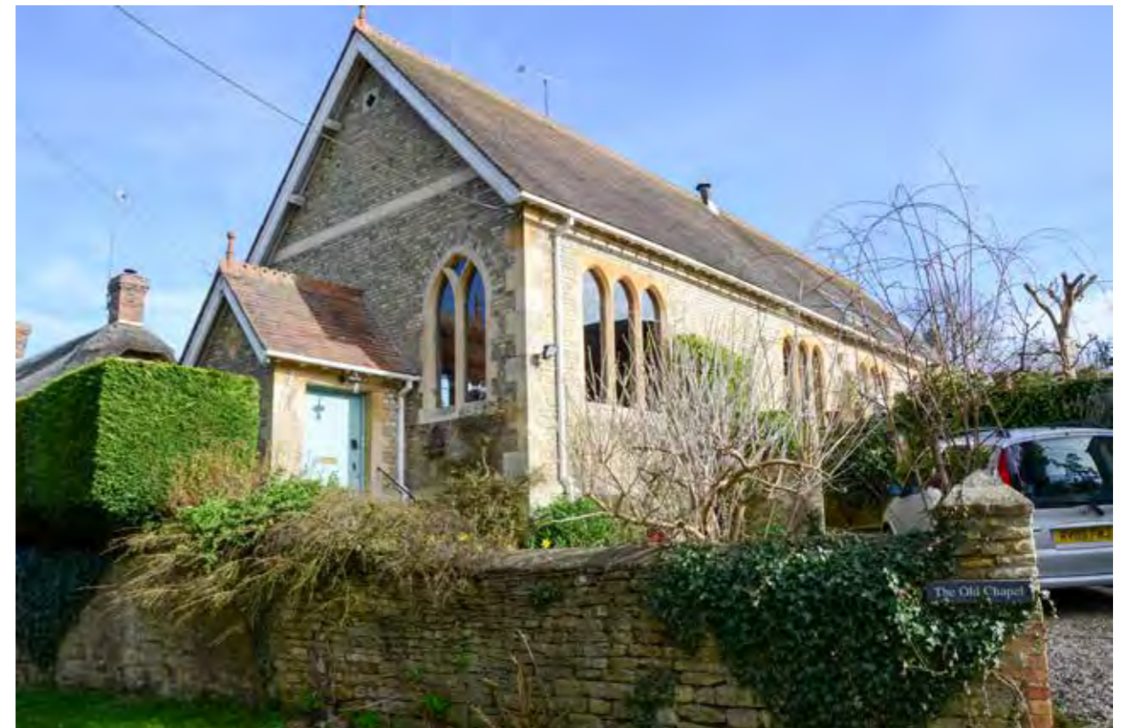
B. Old Chapel, Mill Lane
