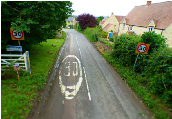
Entry to Somerton marred by road markings
