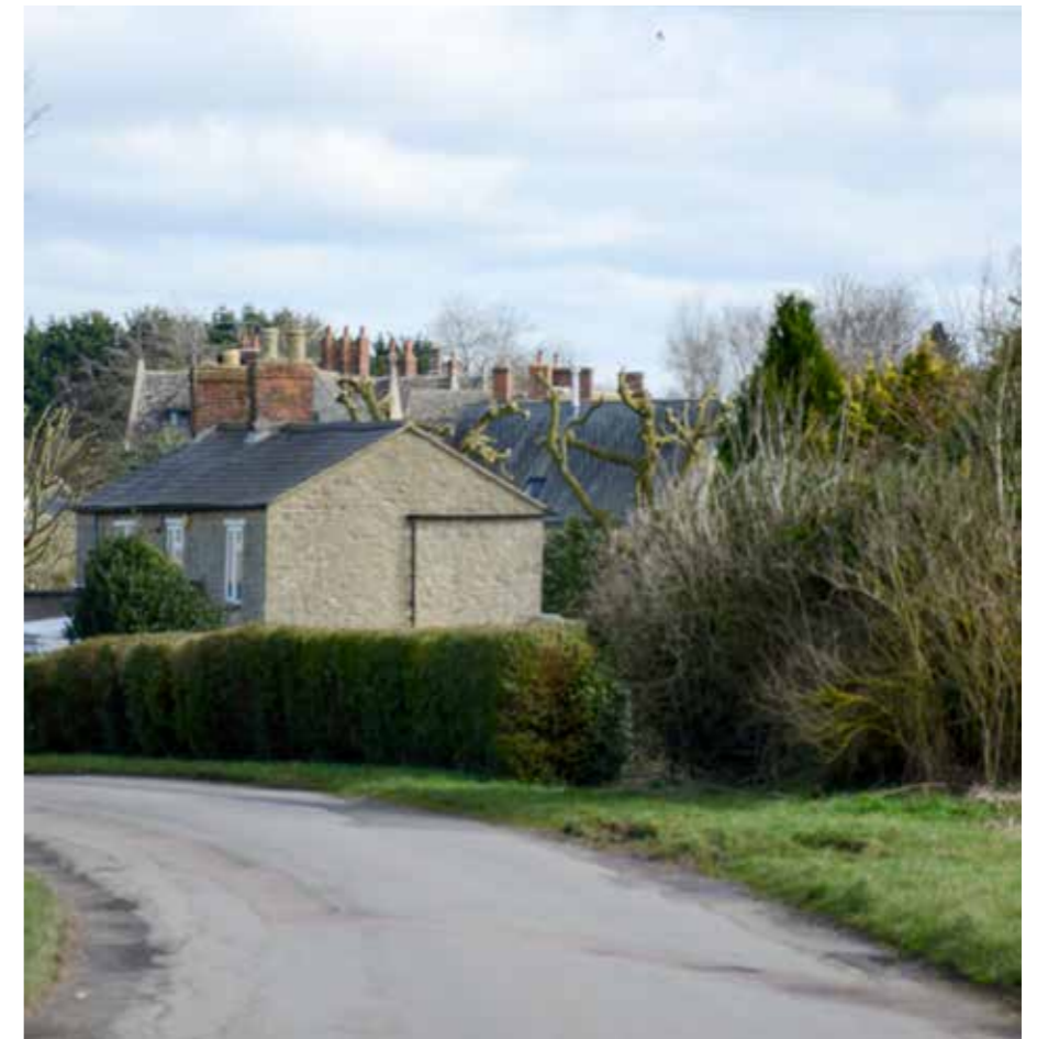
Chimneys and roofscape of the village on the approach from the west
