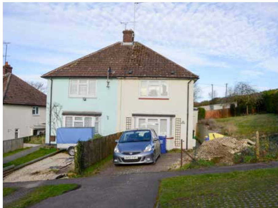
Housing and front gardens that are not sympathetic to the local vernacular
