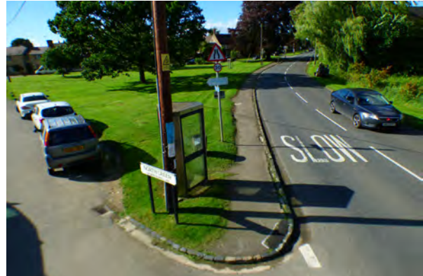
The street through North Green could become part of Kirtlington
